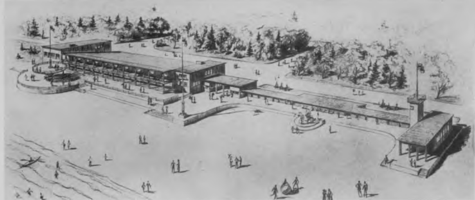
PÄRNU: THE NEW CAFÉ ON THE BEACH (UNDER CONSTRUCTION). MS
