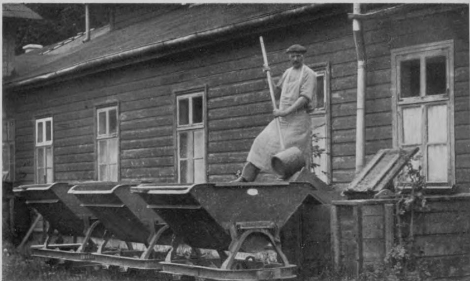
KURESSAARE: DISCHARGING FRESH MUD INTO THE MUD-TANKS.
